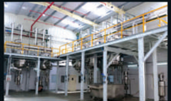
Spice Oils Distillation Plant
