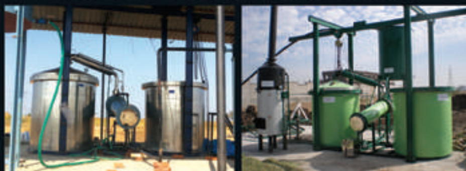
Field Level Distillation Plant ( SS & MS )
